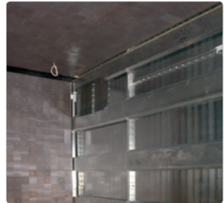
Structure for the installation of ferrite absorbers
